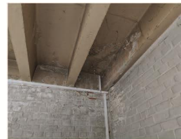
Fig 65: Degradation due to moisture.
