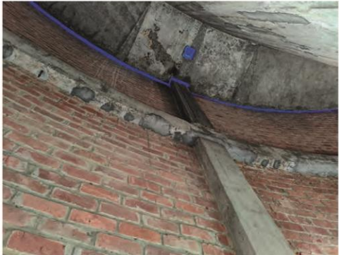
Fig 6: The repairwork on the tank and mantle inside the superstructure.
