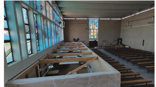
Fig 89: Additional volume set-up in hempcrete.
