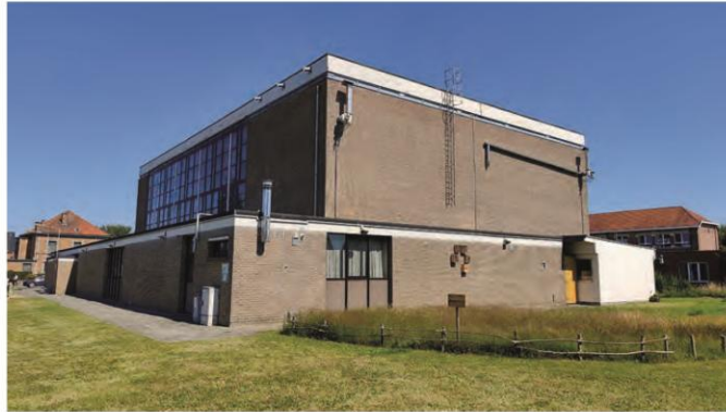
Fig 84: Numerous additions like heating outlets, air ducts, chimneys, rainwater drainage. Annex building in white.
