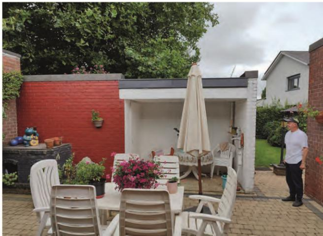
Fig 113: The patio's were also provided with additional storage space and shelter.
