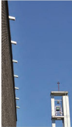
Fig 85: Bell tower and replacement of the concrete gargoyles with steel ones.
