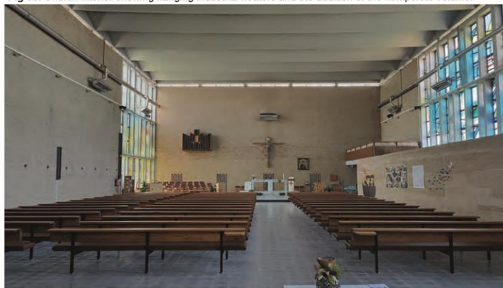
Fig 86: Church interior showing hanging industrial heaters and the addition of the hempcrete volume.
