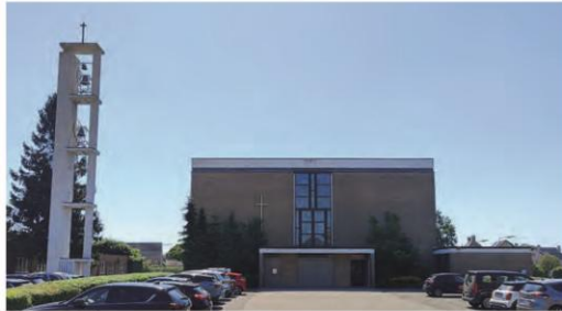
Fig 83: Bell tower and church entrance. Difference in roof height at the eave of the lower volumes due to insulation.
