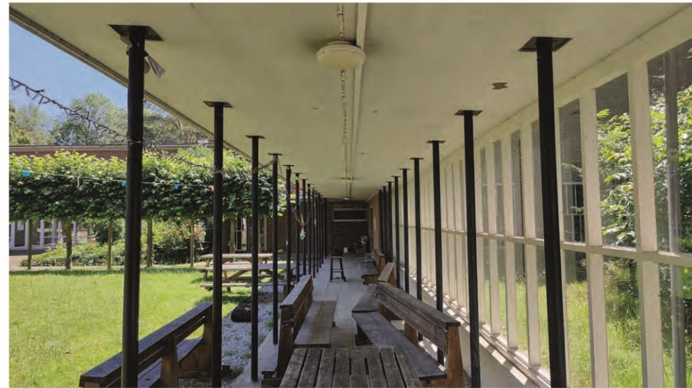
Fig 209: View underneath the outside canopy, leading to the chapel.
