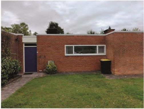
Fig 111: Numbers 45 and 48 are among the most original units remaining. Including original single-glazed windows and front door in typical blue.
